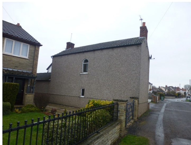
Plate 19: View of 6 Marsh Road looking east
