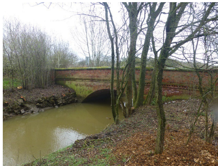
Plate 13: View of bridge adjacent to Dirtness Cottage
