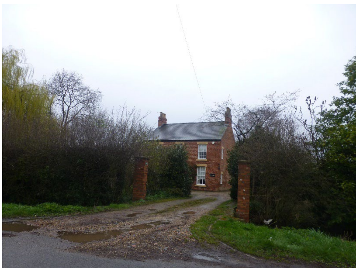
Plate 45: View of Meaburns, looking east
