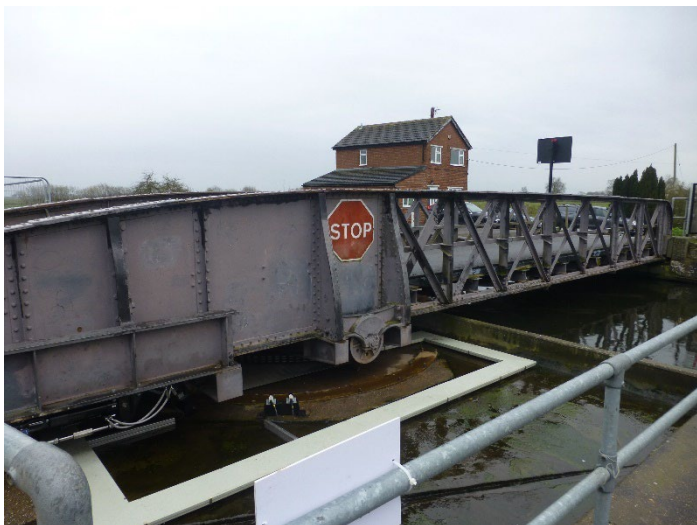
Plate 40: View of the bridge looking south-east
