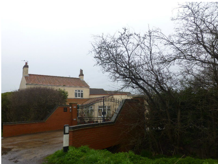
Plate 47: View of The Willows, looking north-east
