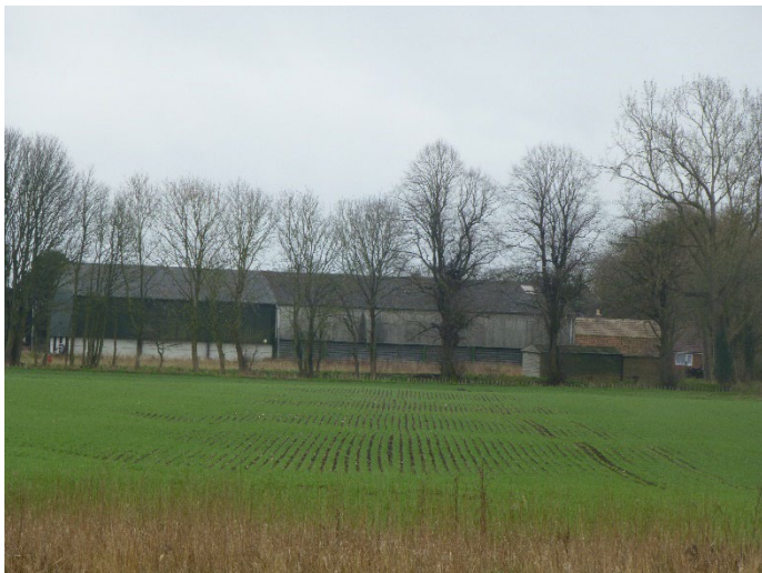
Plate 22: View of Belton Grange looking south
